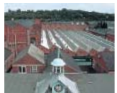
NSK Newark Plant
